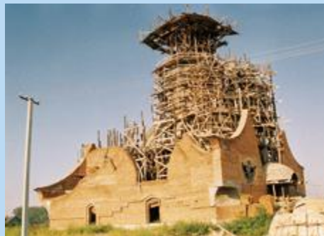
Church under construction
